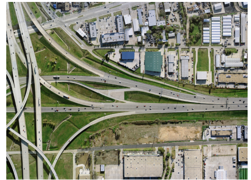
A color aerial photograph highlights the Lyndon B. Johnson Freeway in Dallas.
